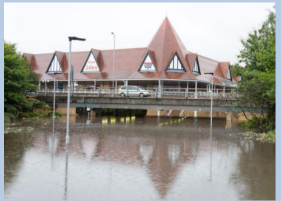
Figure 1 Purley Cross underpass (Croydon,2015)
